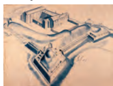
Under construction. The castle seen from SW. A drawing made by the master builder Hans Fleming in 1605, showing bastion Gustavus in the background. The buildings of the former friary are still easily recognizable. © The Military Archives Sweden
