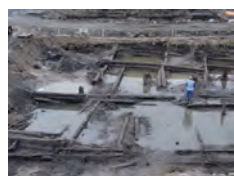
The Moats. Timber structures used for stabilizing landfill in the late 17th century. Excavated in 2004. Photo: Jönköping County Museum
