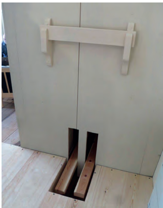
Kalkanttrampor till bälgverket. Foto: R. Gullbrandsson. Pumping pedals for the bellows.
