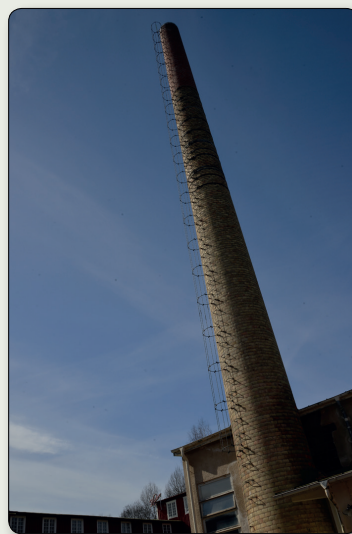
The industrial chimney was originally constructed in yellow brick and later extended in red brick. Photo: Jönköping County Museum.
