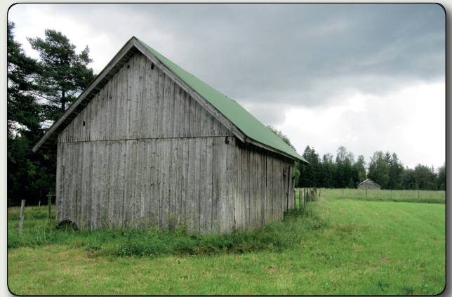
Field barn with timber frame and vertical boarding. Photo: Jönköping County Museum.
