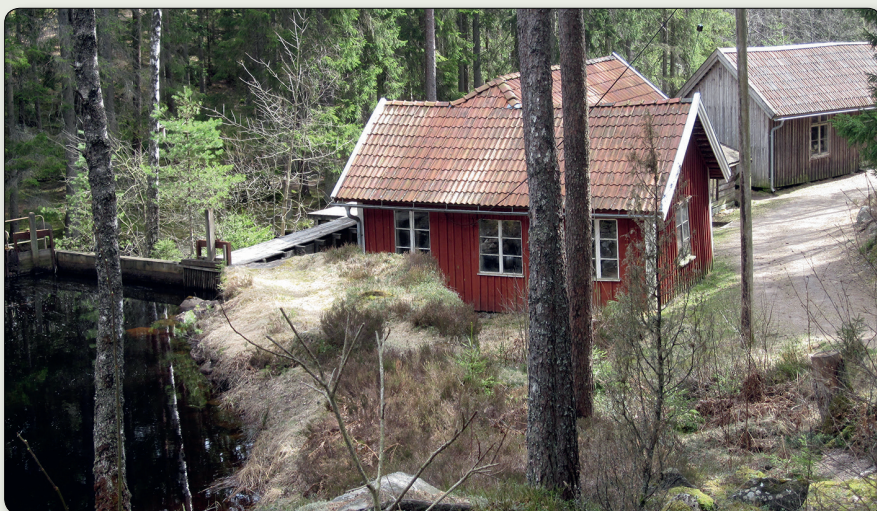
The seemingly simple buildings contain both history and technology. In the foreground, the Andersfors industrial building from 1908 in its original position. Behind, you see a glimpse of Lill-Andersa's workshop, which housed Gnosjö's first hairpin factory and a smithy. Photo: Jönköping County Museum.
