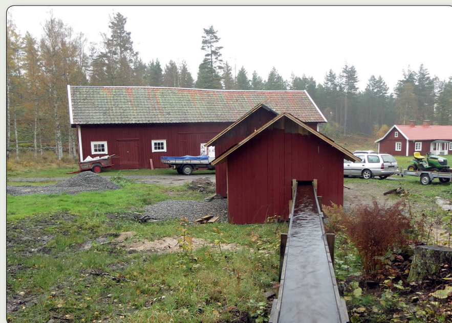
Water is led from the small stream, via a simple wooden chute, to the wheelhouse. Photo: Jönköping County Museum.
