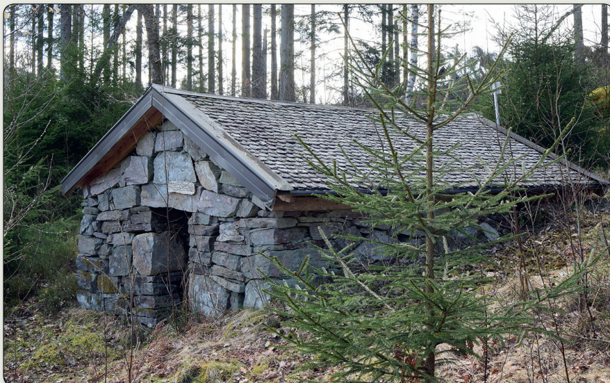
The small stone cellar was used for storing explosives. The roof is made from local slate. Photo: Jönköping County Museum.
