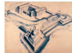
Under construction. The castle seen from SW. A drawing made by the master builder Hans Fleming in 1605, showing bastion Gustavus in the foreground. The buildings of the former friary are still easily recognizable. © The Military Archives Sweden
